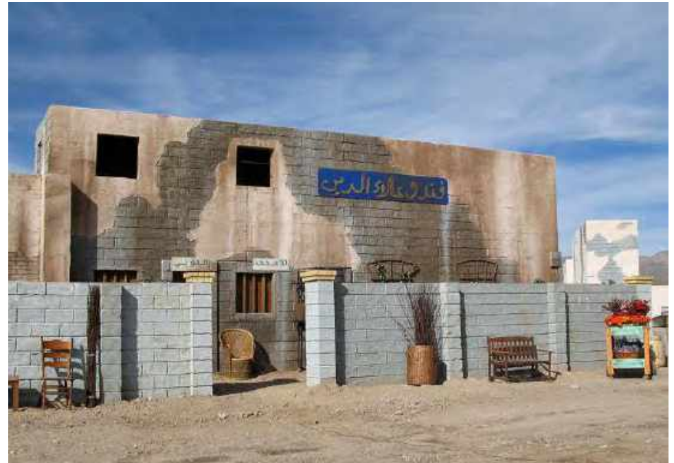
Concrete Masonry Unit (CMU) Compound Wall
