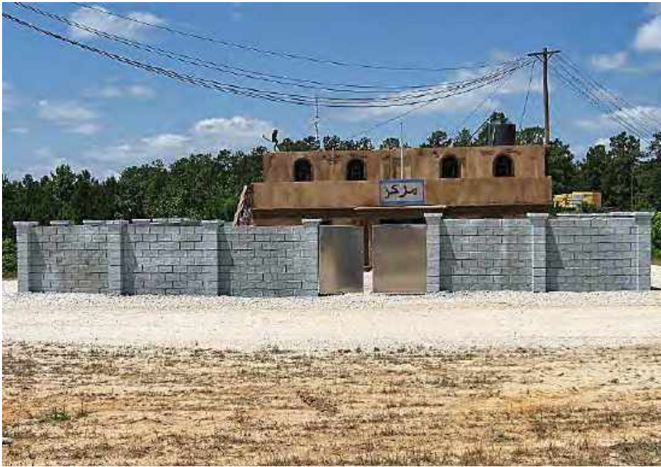
CMU Compound Wall with Vehicle Gate
