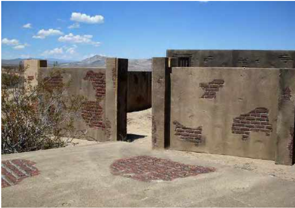
Mud over Compound Wall
