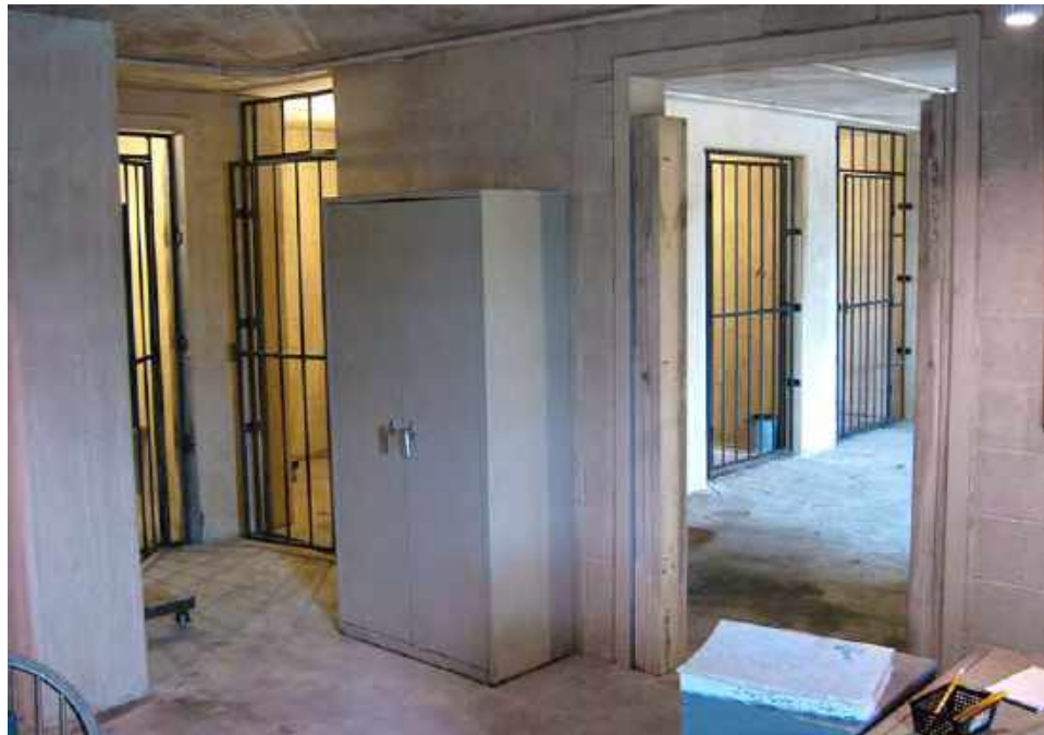
Jail Cell Complex
