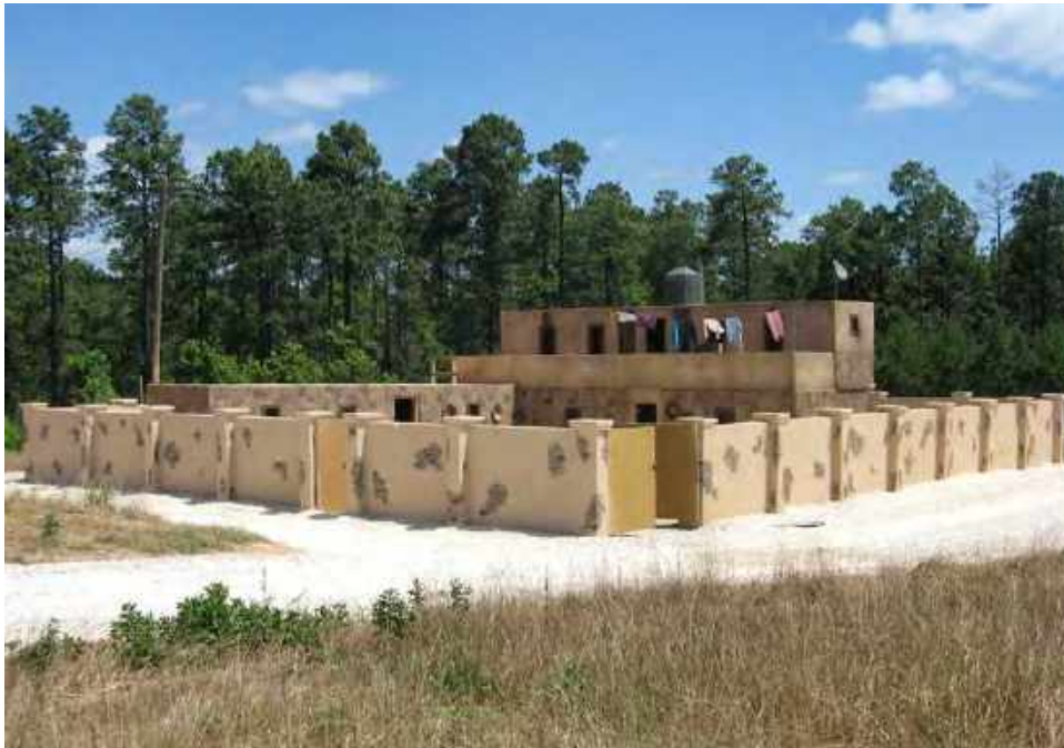
Mud over Brick Compound Wall with Vehicle and Personnel Gates
